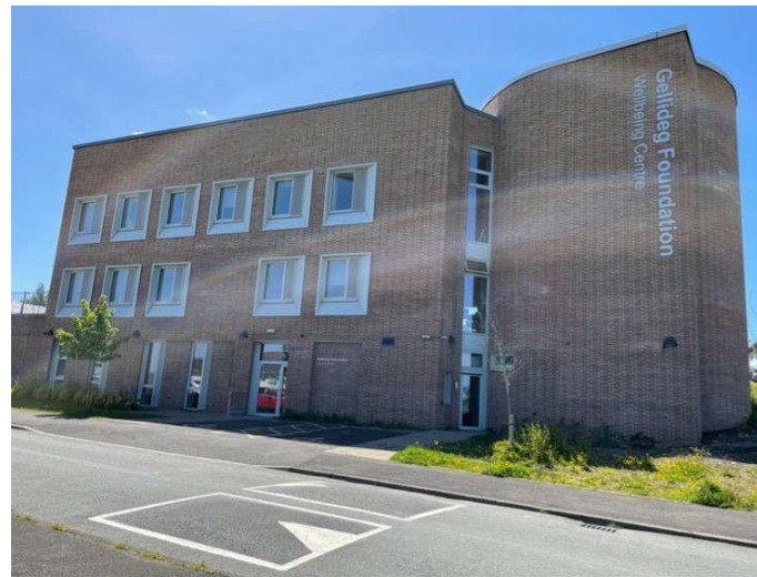
Fig. 2 / Entrance to the hall and entrance to the youth wing, off Lansbury Road.
