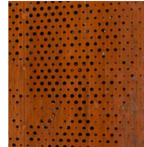
Perforated metal shutters
