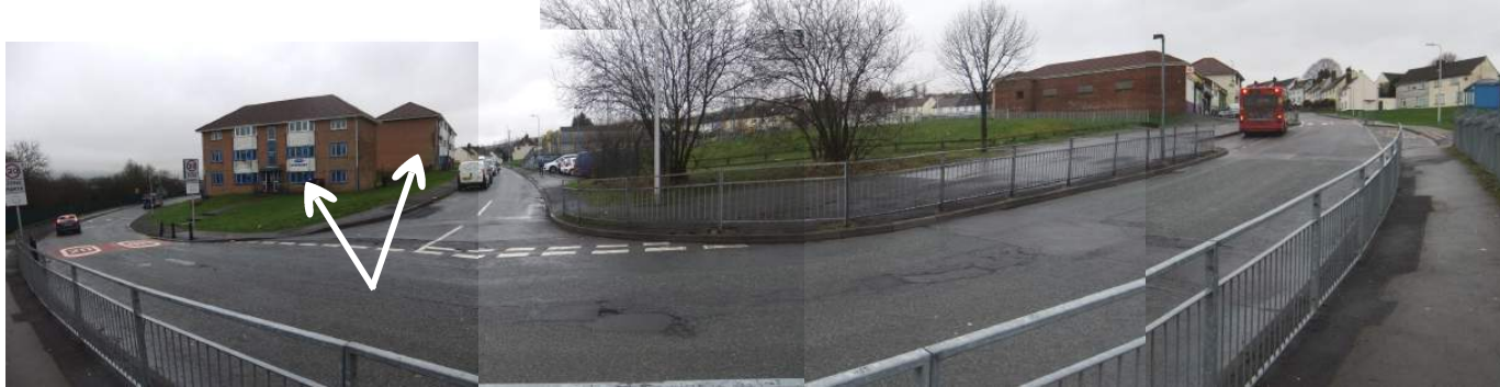
P4. View from junction of Lansbury Road with Heol Tai Mawr - building marked will be demolished & replaced with MVH Office and car park
