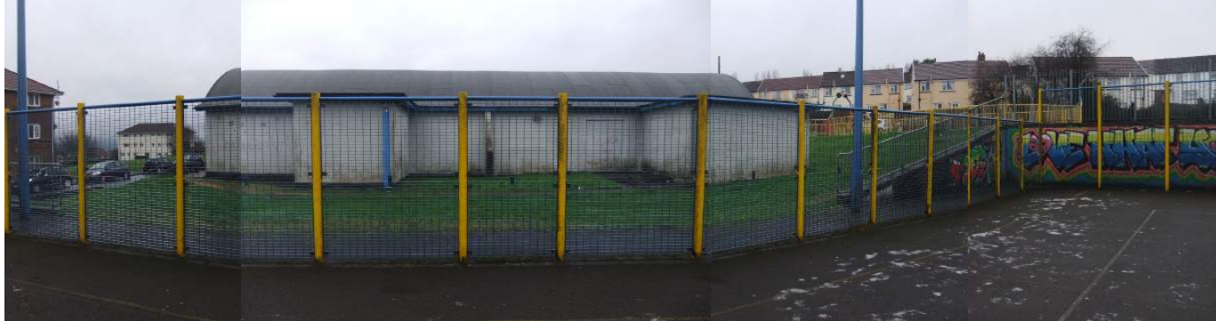
P5. View from MUGA to side elevation of St Lukes Church
