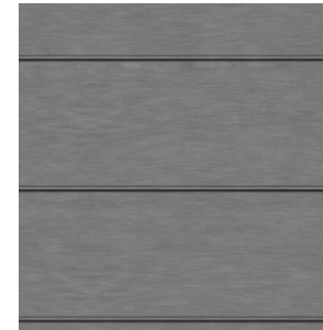
Metal standing seam roof
