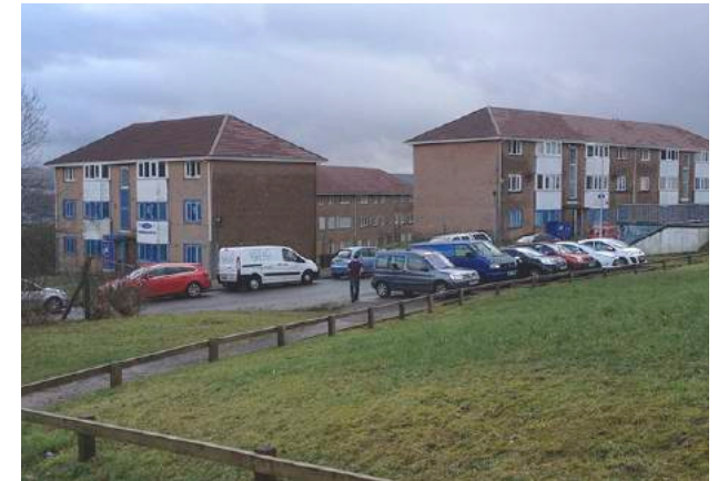
Flats currently occupied by the Foundation
